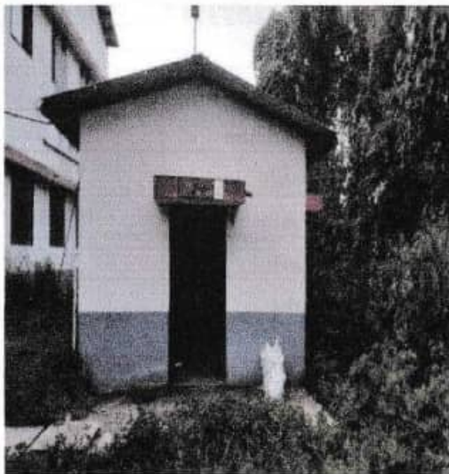
Figure 3. Sewage treatment plant
