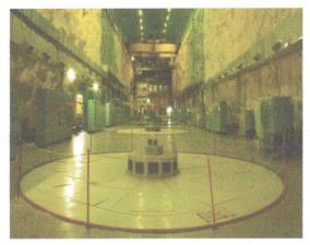
Varahi Hydro Power Plant is located near Hosangadi in the Udupi district of Karnataka in India. The power project is commissioned in 1993 with an approved and installed capacity of 460 Megawatt. The type of Hydro Electric Project is major as the capacity is greater than 25 MW and the type of Powerhouse is underground. The source of water for the generation of power is Varahi River. The power plant is owned by State Government and the operating organization is Karnataka Power Corporation Limited.
