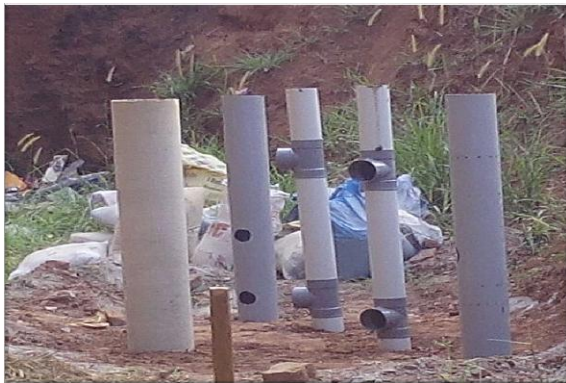
Fig. 1 Installation of different Pipes.
